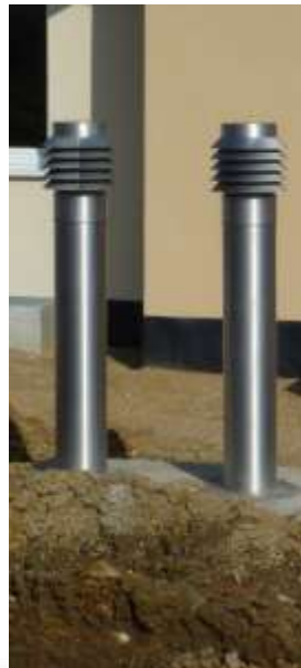
Part of the ventilation system; intakes, air tempering through buried pipes, exhaust, HRV and distribution
